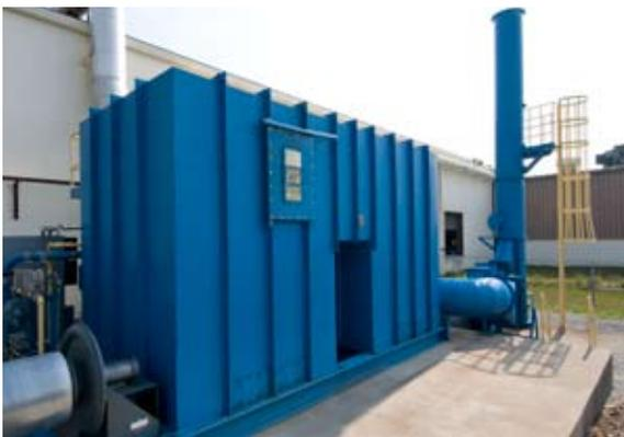
*ThermaGrid RTO system (volume flow: 13,000 scfm) controlling VOCs from a paint oven.*
