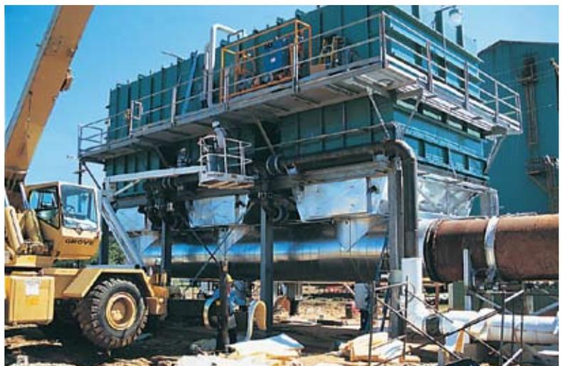
*McGill can provide total system responsibility including field installation. Here the final insulation and lagging is being completed for a three-bed ThermaGrid RTO that controls emissions from a large particle board press.*
