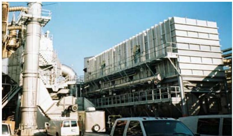
*McGill provided its wet electrostatic precipitator upstream of its ThermaGrid RTO to control particulate and d-limonene emissions from a citrus peel dryer.*
