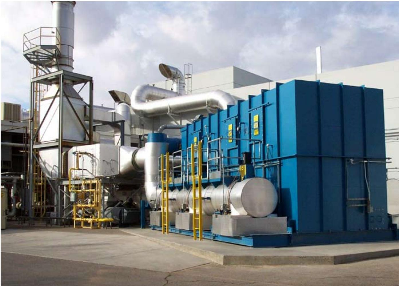
*ThermaGrid RTO system (volume flow: 15,500 scfm) controlling xylene emissions for an electronics manufacturing application.*
