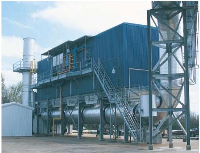
*ThermaGrid RTO system for a fiberboard dryer and preheater (volume flow: 90,000 scfm) controls hydrocarbons, formaldehyde, formic acid, carbon monoxide, aerosols, and wood fiber emissions.*
