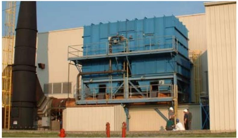
*ThermaGrid RTO system (volume flow: 50,000 scfm) controlling formaldehyde and phenol emissions from a fiber glass curing oven.*
