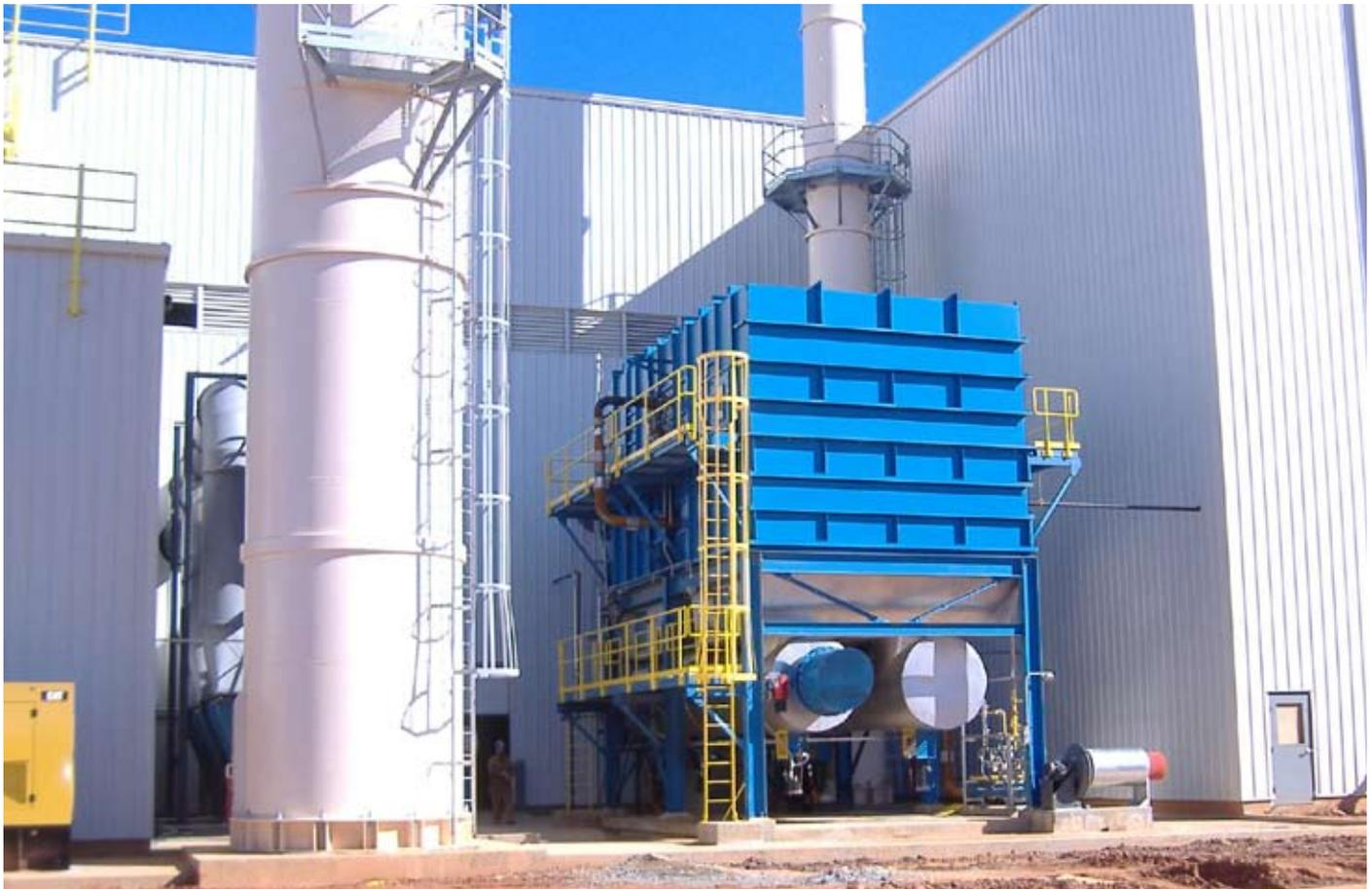
*McGill's modular design weighs less and requires a smaller footprint, allowing the RTO to be installed in tighter spaces than conventional systems.*
