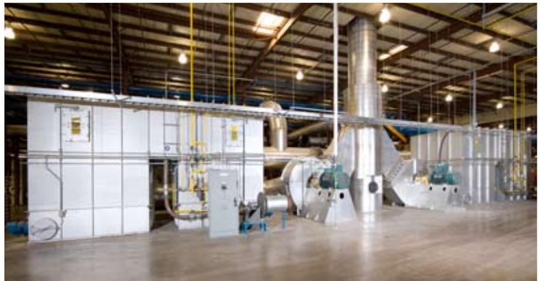
*Two ThermaGrid RTO systems (volume flow: 31,000 scfm each) installed inside a plant and controlling organic binders, formaldehyde, and phenol emissions for a fiber glass manufacturing process.*
