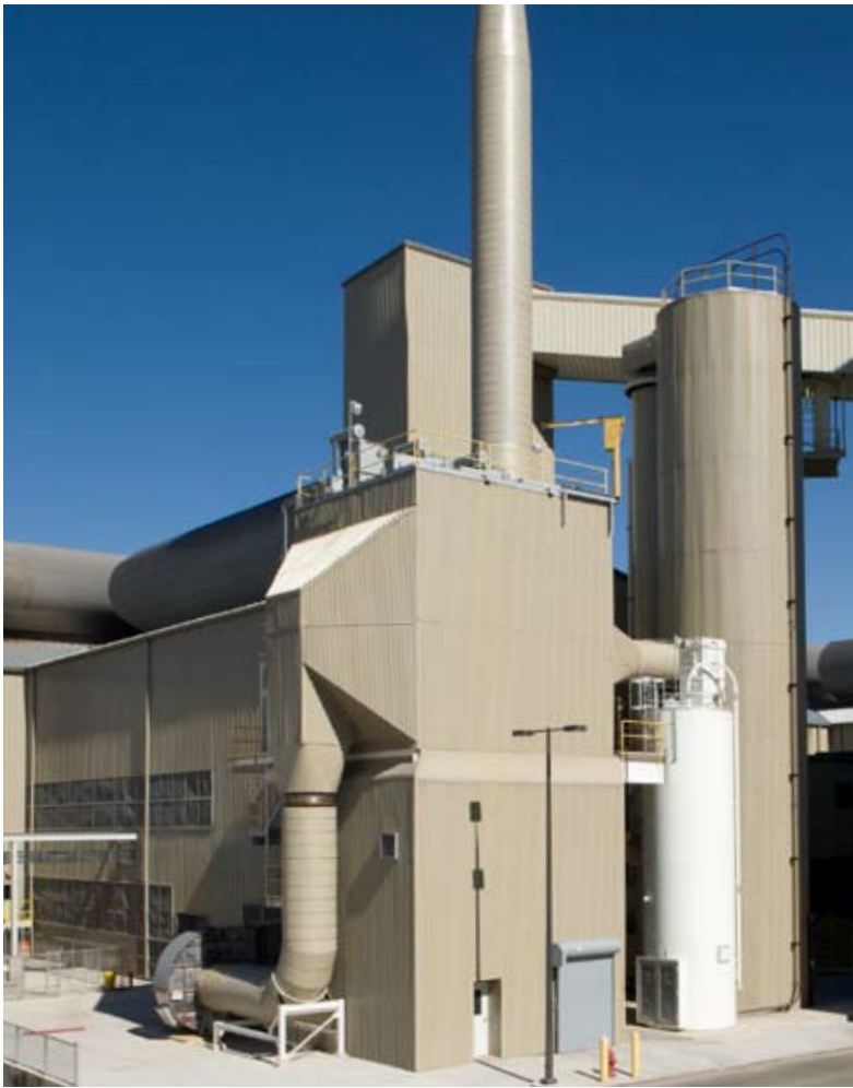
McGill supplied this Trona-dry scrubber and dry electrostatic precipitator system to control SO 2 and particulate from a container glass furnace.
