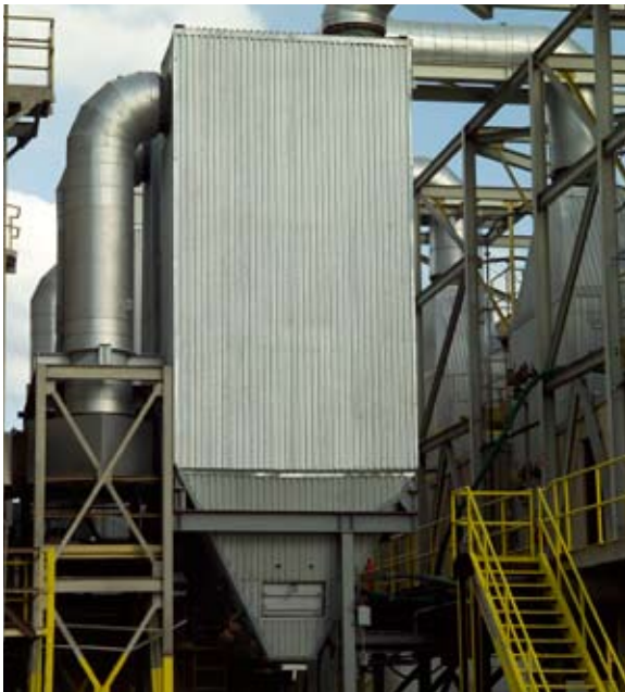
Three McGill reaction chambers with lime injection systems control HCl and SO 2 from three MSW incinerators.
