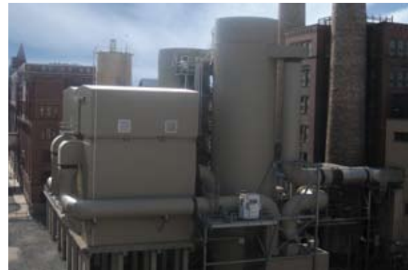
Two spray-dry scrubbers and fabric filter systems controlling SO 2 , HCl, Hg, and particulate from four coal-fired boilers.
