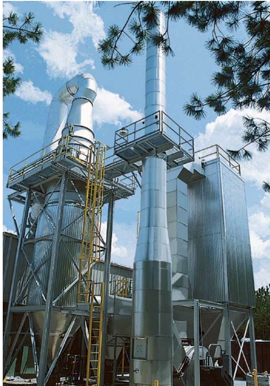
This turnkey system uses evaporative cooling, dry reagent injection, and a fabric filter to control acid gas and particulate emissions from a regional medical waste incinerator. The unique and proprietary cooler inlet duct arrangement was determined by flow modeling to avoid using gas distribution devices in the 2,400°F environment.
