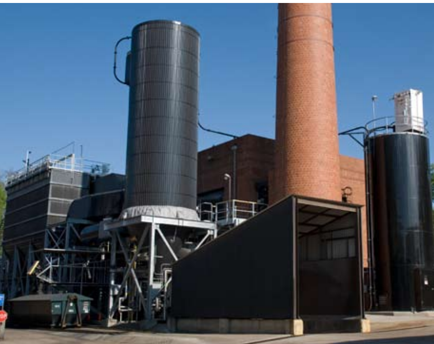
A McGill evaporative cooler and dry lime injection system controlling HCl and SO 2 on a university's coal-fired boiler.
