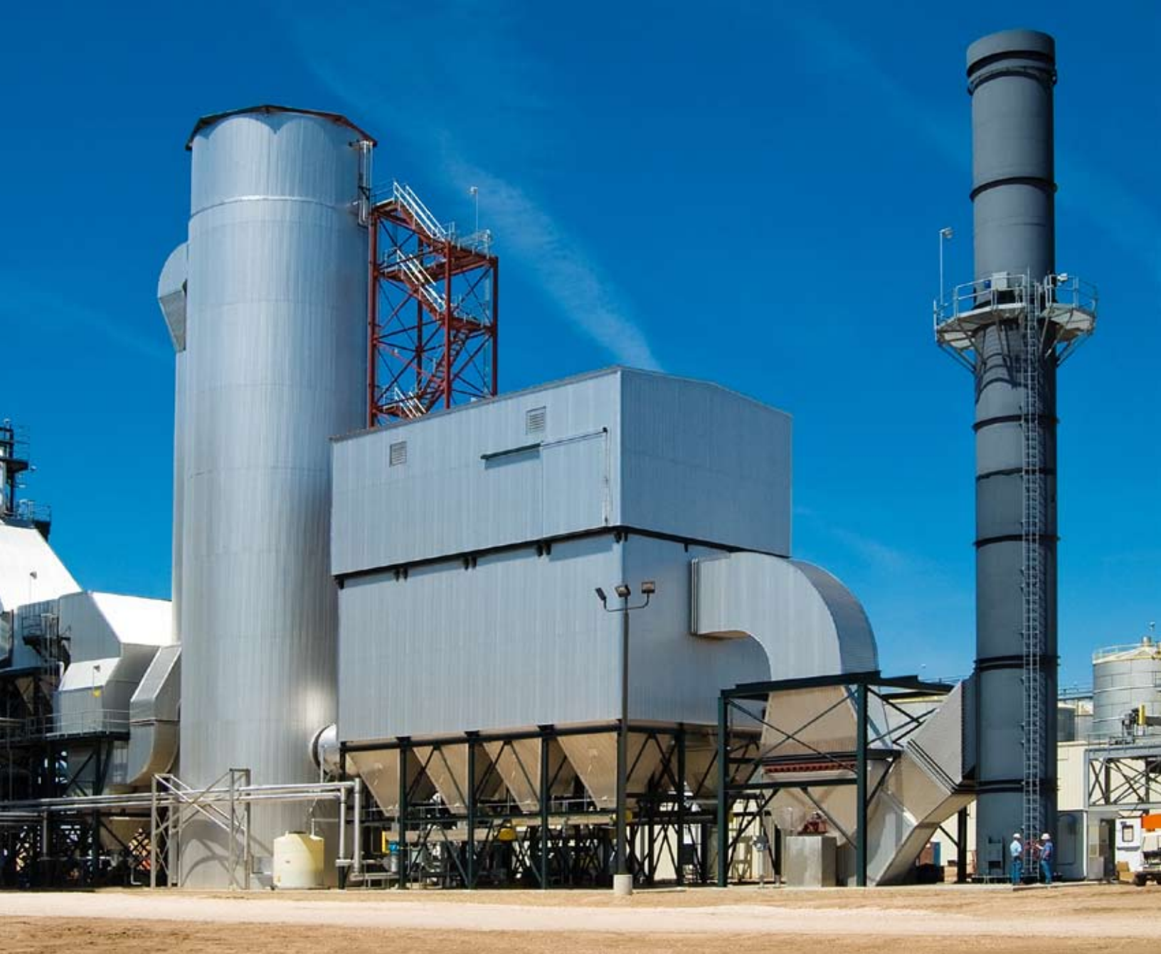
McGill supplied this large (27-foot OD) spray-dry scrubber and eight compartment fabric filter system on a manure-fired BFB boiler to control HCl, SO 2 , and particulate.
