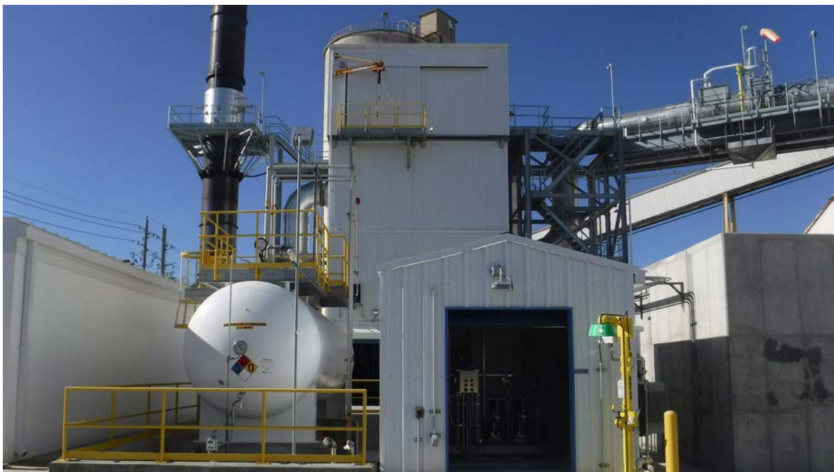
McGill 4 Module Catalytic Filter System, controlling particulate and NO x on a container glass furnace.
