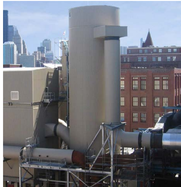
4) The completed system.
