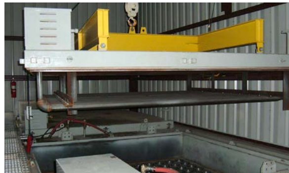
An overhead crane is used to remove the top lids from the catalytic filter’s modules to provide easy access to the collection filters.
