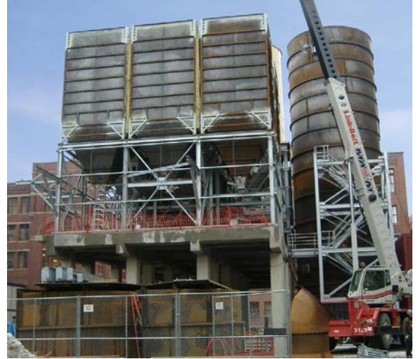
2) With the foundation work completed, and the structural steel erected, the last of the modules for this catalytic filter system is lifted into place
