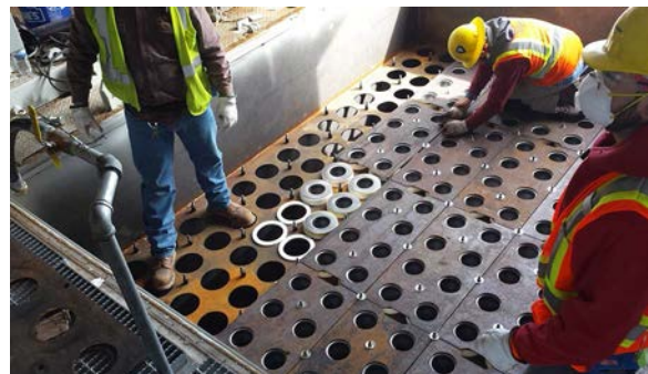
With the top lid removed, filter maintenance can be performed in a safe, ambient air environment.
