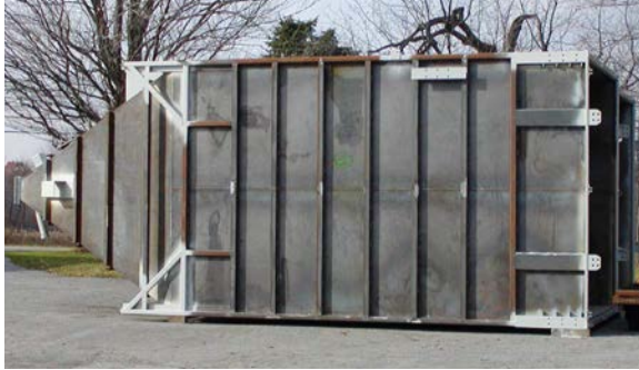
1) A catalytic filter module delivered to the jobsite and ready to be rigged for lifting.
