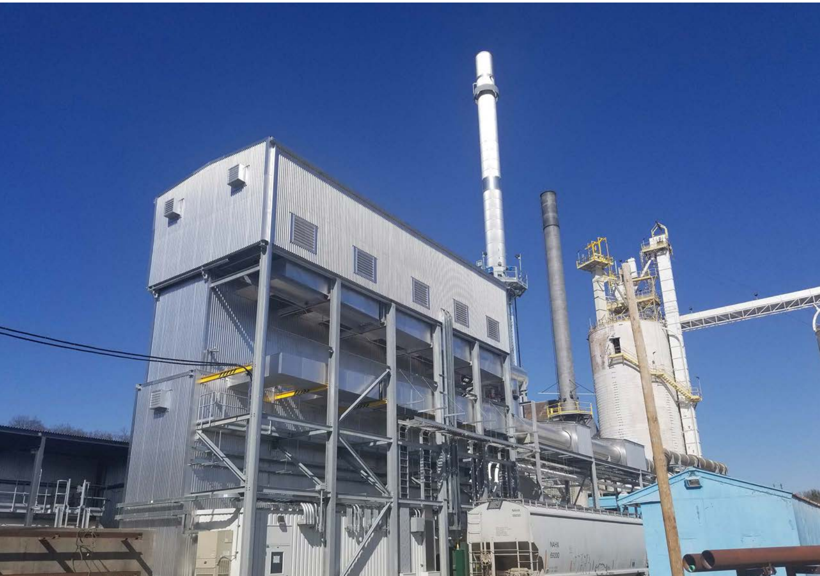
McGill 5 Module Catalytic Filter System, controlling particulate, SO x and NO x on a container glass furnace.
