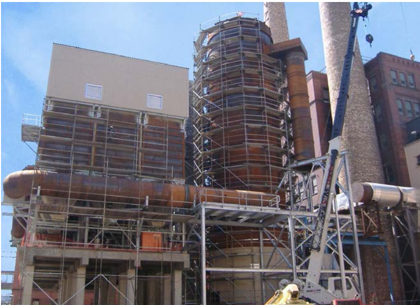
3) Once the modules, hoppers, scrubbing tower, and manifolds have been erected, insulation is applied prior to the installation of the exterior siding.
