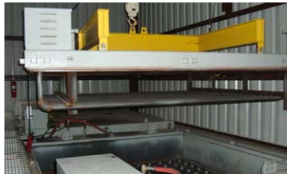
An overhead crane is used to remove the top lids from the fabric filter’s modules to provide easy access to the collection bags.
