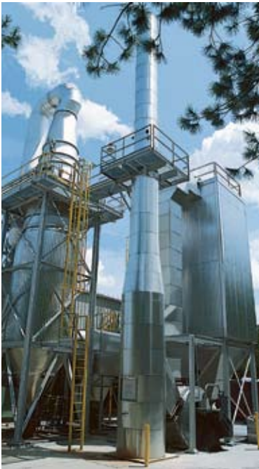
This turnkey system uses evaporative cooling, dry reagent injection, and a fabric filter to control acid gas and particulate emissions from a medical waste incinerator.
