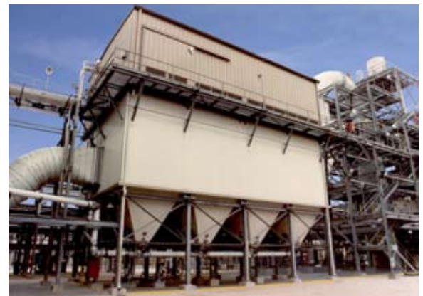
An eight-module fabric filter controls emissions from a rotary kiln incinerator that burns hazardous waste.
