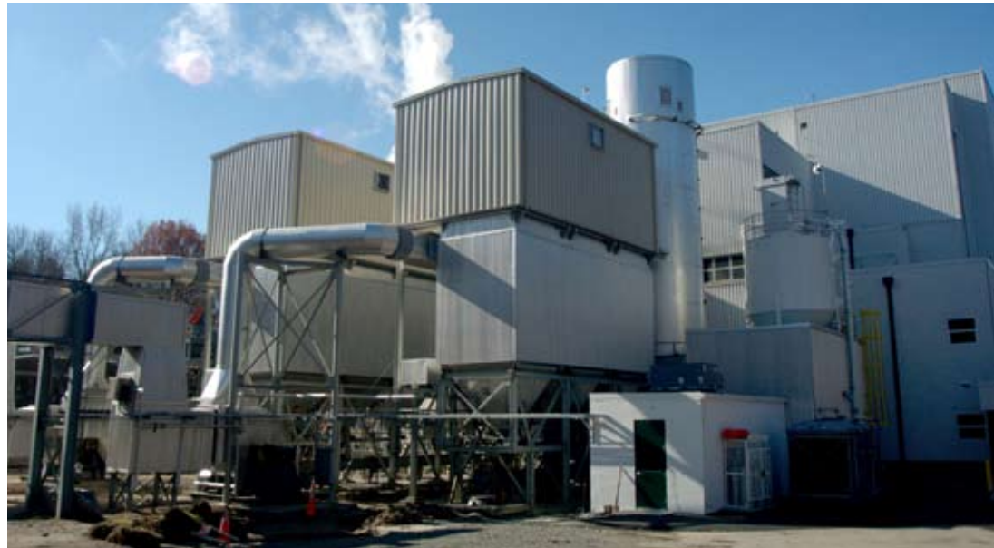
A pair of spray-dry scrubbers, each with its own three-module fabric filter, control HCl, SO 2 , and particulate from two 100-tons per day municipal solid waste incinerators.
