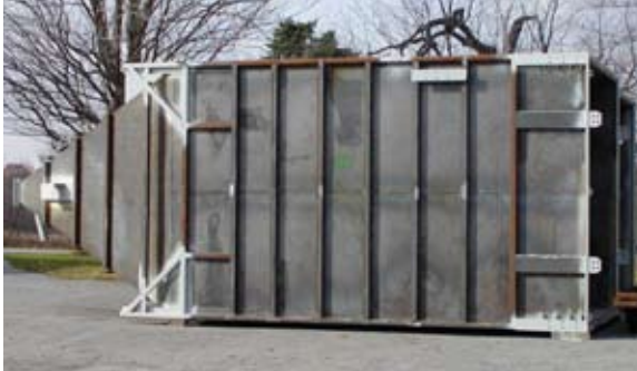
A fabric filter module delivered to the jobsite and ready to be rigged for lifting.
