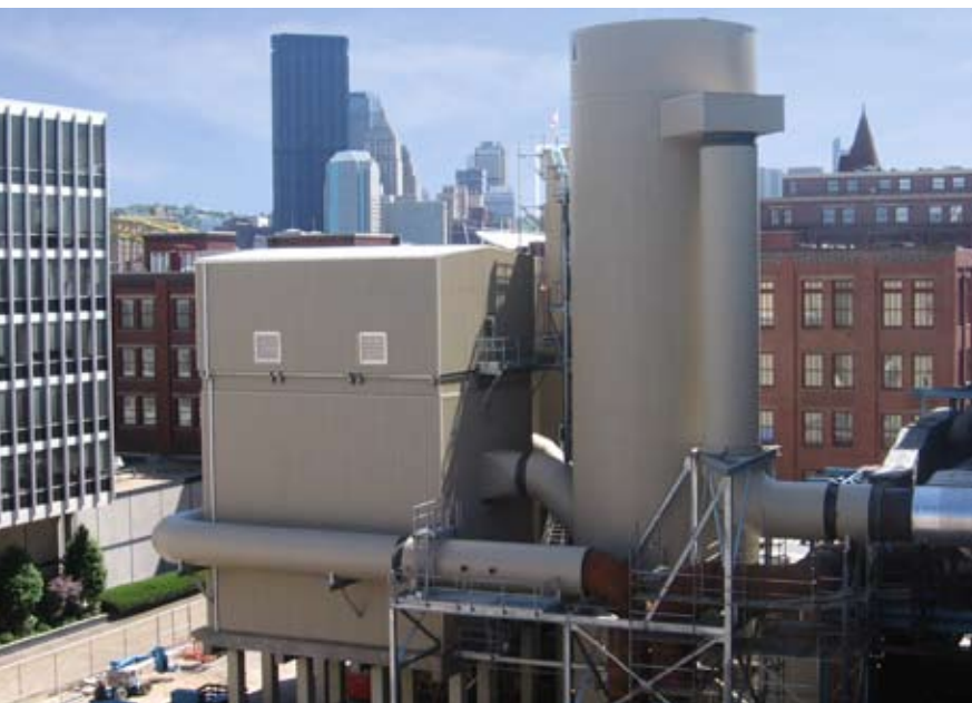
The completed system, comprised of two spray-dry scrubbers and two fabric filters, controls SO 2 , HCl, Hg, and particulate from four coal-fired boilers.
