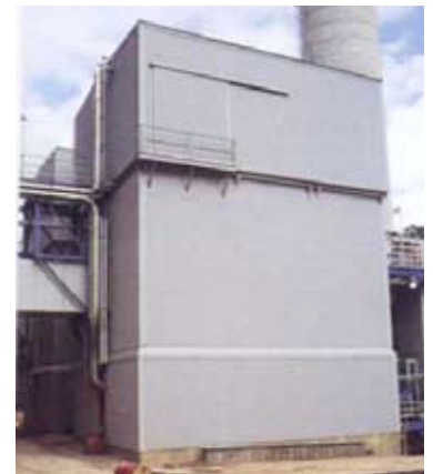
Two six-module fabric filters control the emissions from a coal-fired, circulating fluidized-bed boiler.
