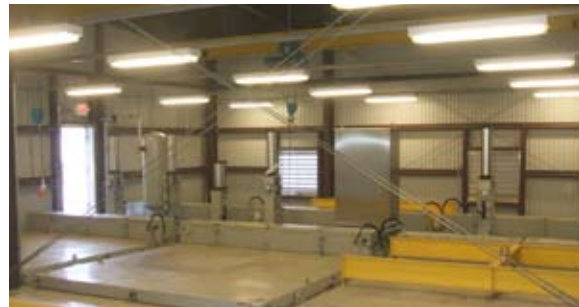
A view from inside the penthouse atop the fabric filter system.
