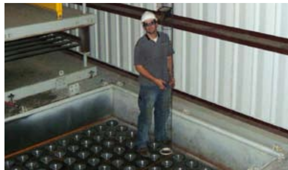
With the top lid removed, bag maintenance can be performed in a safe, ambient air environment.
