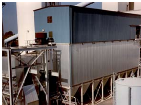
A sixteen-module fabric filter system controls particulate from a 650,000 lb/hr circulating fluidized-bed boiler that burns anthracite culm.
