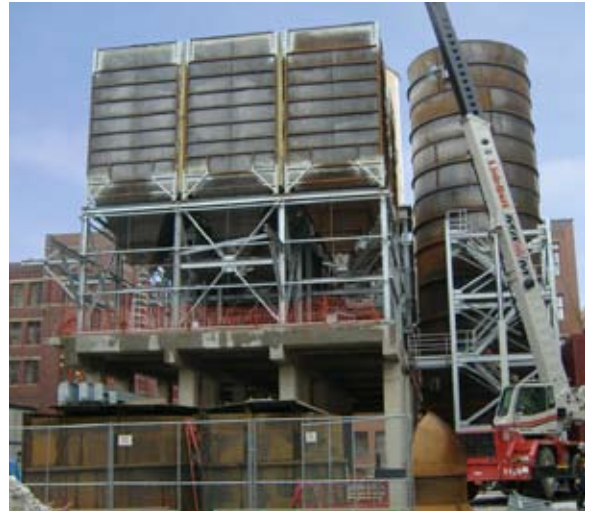
With the foundation work completed, and the structural steel erected, the last of the modules for this fabric filter system is lifted into place.
