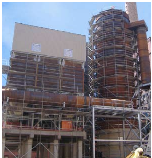
Once the modules, hoppers, scrubbing tower, and manifolds have been erected, insulation is applied prior to the installation of the exterior sheathing.
